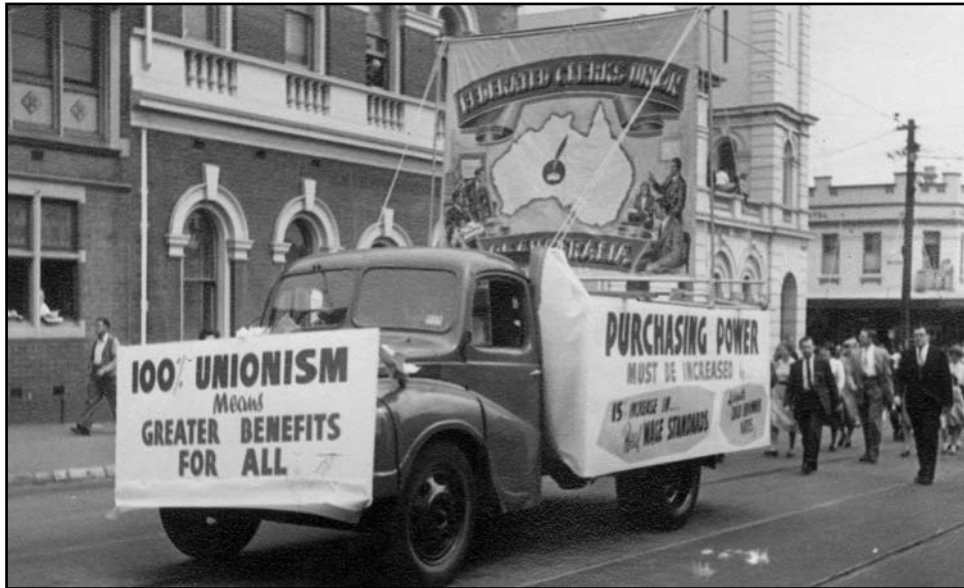
Labor Day Procession – 6 October 1958, near Redfern Post Office
